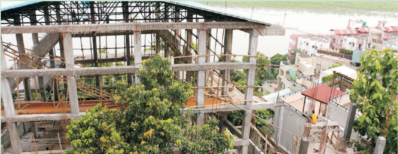
Jubilee Memorial Hall work in progress
